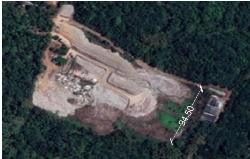
Figure 2. Location of the Retaining Wall
