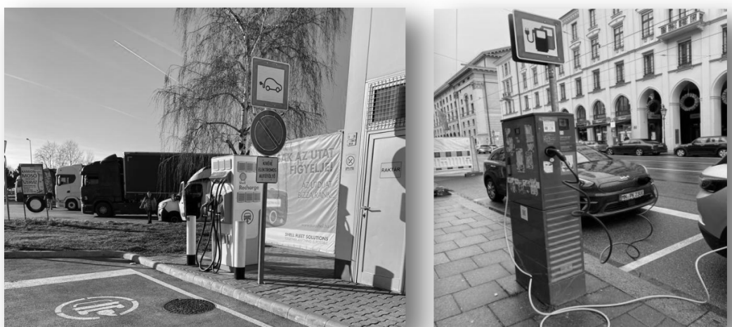
Figure 1 SPKLU without shelter with waterproof IP
