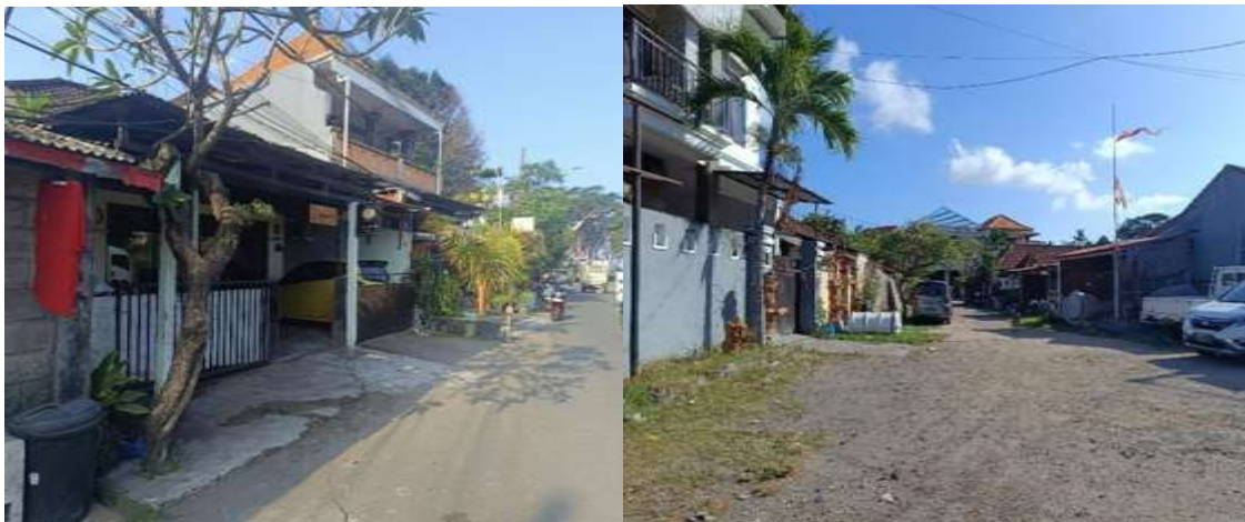
Figure 10. The Condition of Affected Residential Areas Prone to Liquefaction Disasters in Serangan Village Source: Survey Documentation
