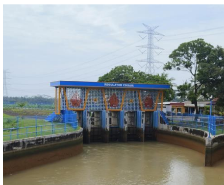
Figure 2. Cihaur Dam Source: Personal Documents
